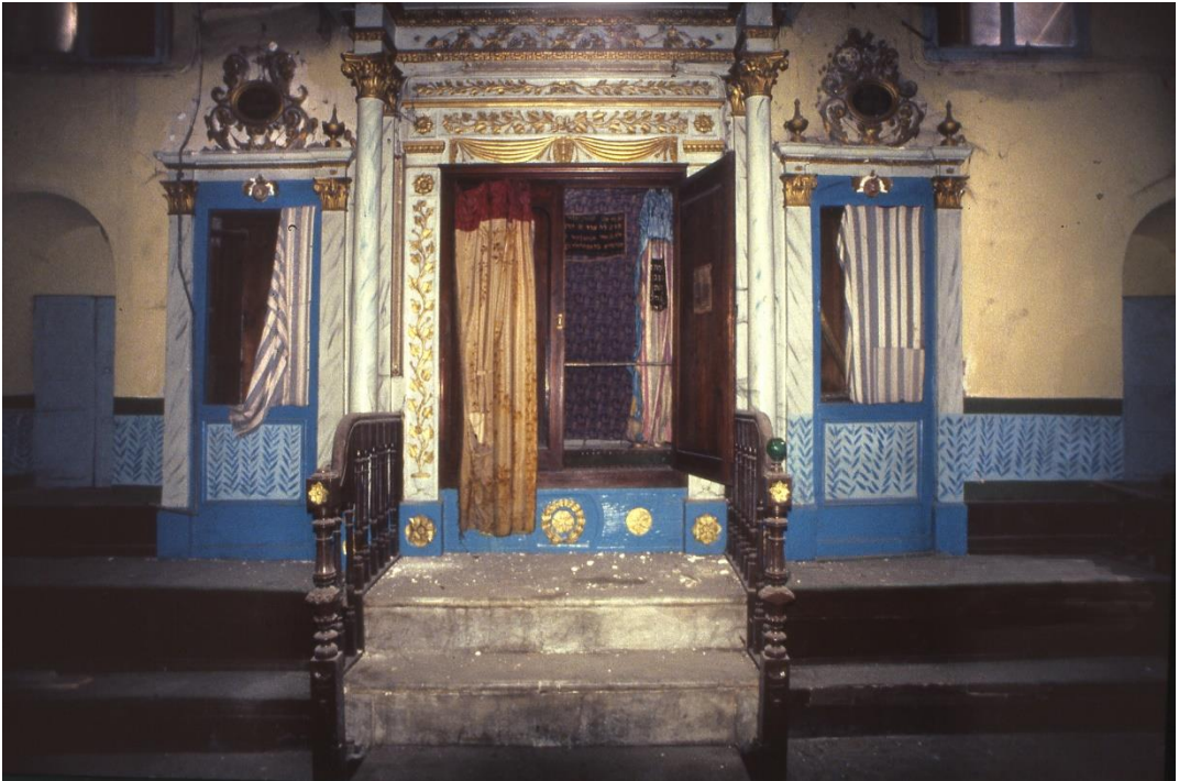
Hevra Synagogue before it collapsed
